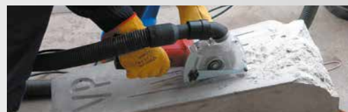
MINI ANGLE GRINDER CUTTING WITH AN EXTRACTION GUARD
