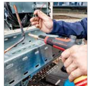
Brazing in refrigeration / air-conditioning technology
