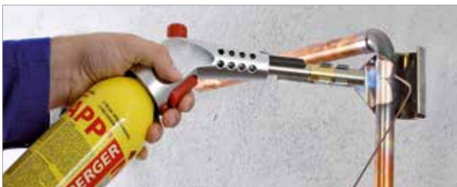
Brazing in gas installation
