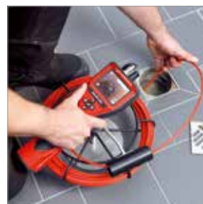
Inspection of floor drains
