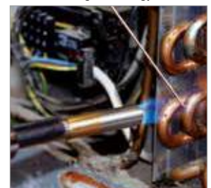
Brazing in refrigeration / air-conditioning technology
