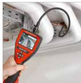
Inspection of hollow spaces
